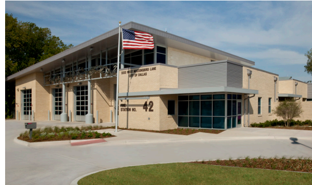
Dallas Fire Station 42, Dallas, TX.
