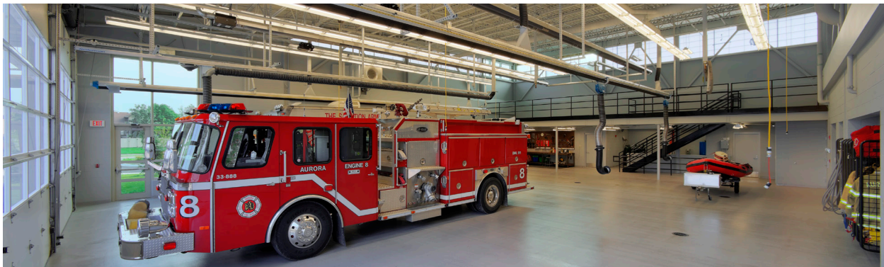
Aurora Fire Station No. 8 and Customer Service Call Center, Aurora, IL.
