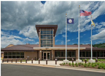
Fair Oaks Police & Fire Renovation and Expansion • Fair Oaks, VA
