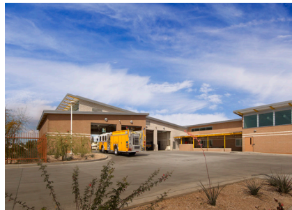
Glendale Fire Station No. 159 • Glendale, AZ
