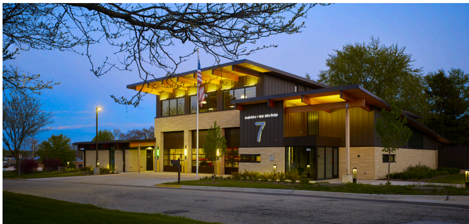
Fire Station No. 7, Aurora, IL
