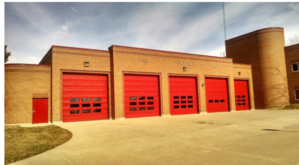
Decatur Fire Stations, Decatur, IL Rich Pruitt, Deputy Fire Chief rpruitt@decaturil.gov / 217.424.2811
