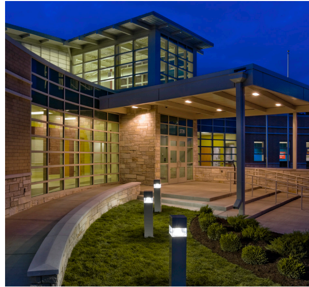
Aurora Fire Station No. 8 and Customer Service Call Center, Aurora, IL.
