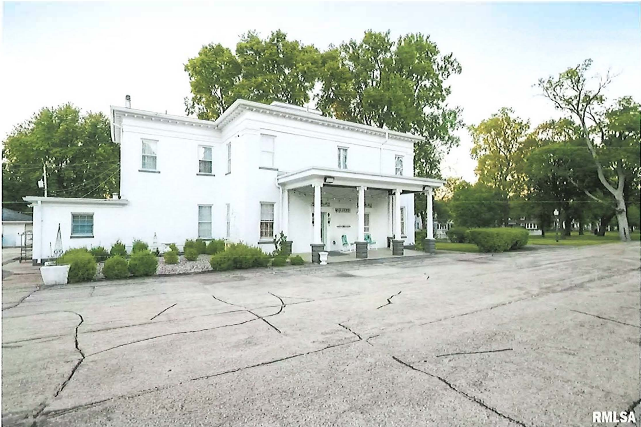
420 Walnut St – East Side Elevation and additional parking
