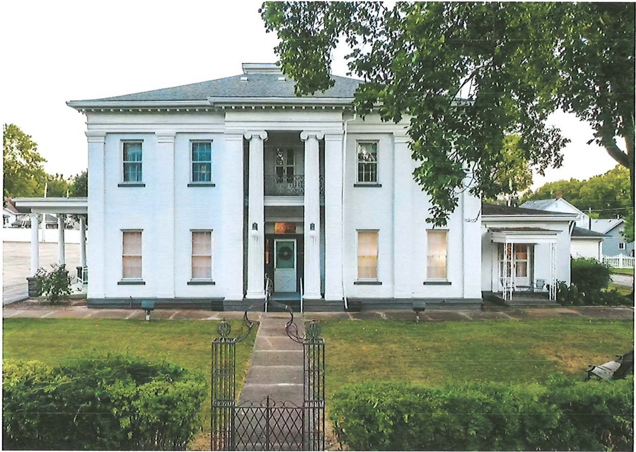
Front Elevation – 420 Walnut St, Pekin, IL – North Elevation
