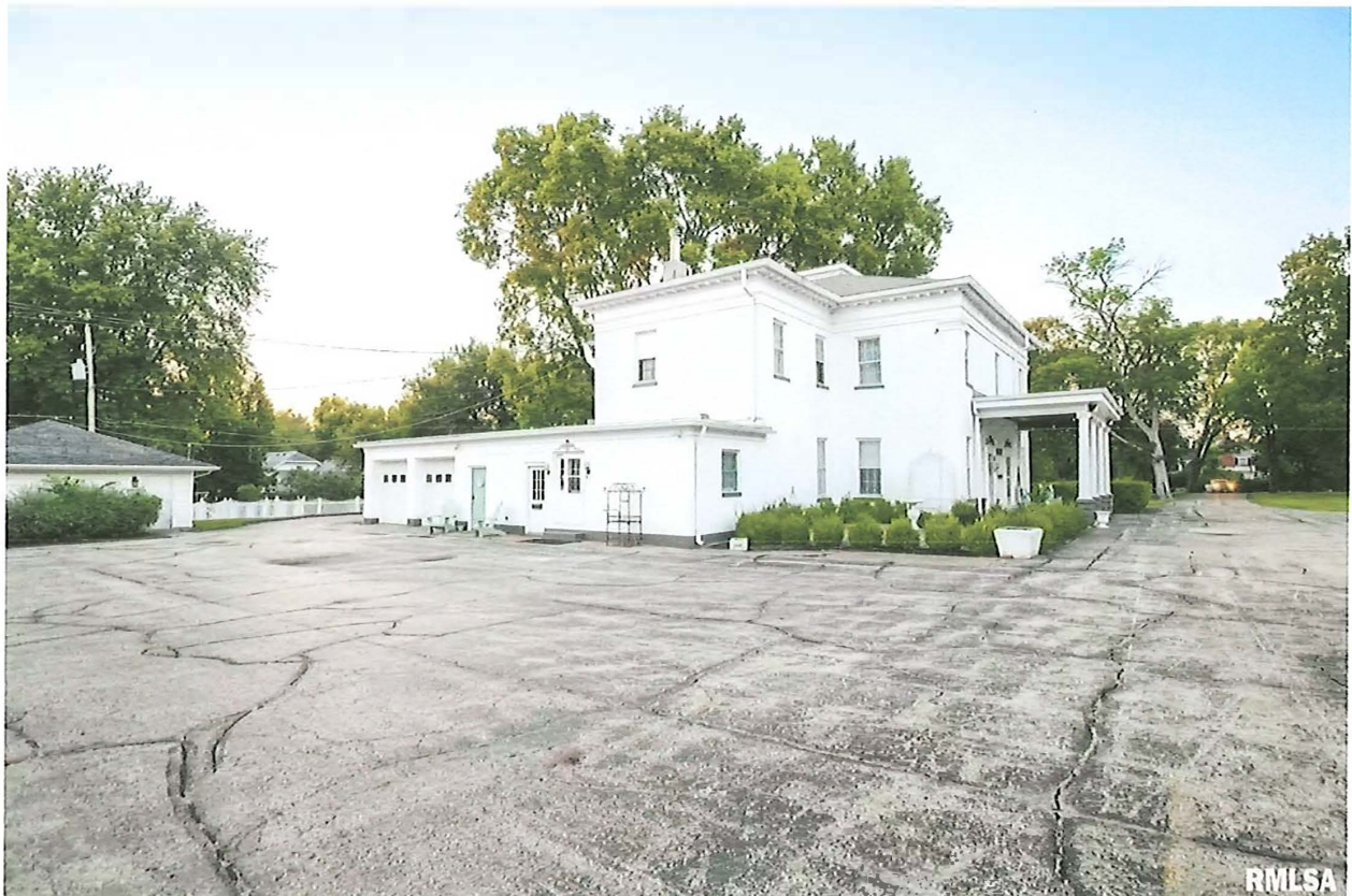
420 Walnut St – South (back) Elevation with Detached Garage and Parking Lot
