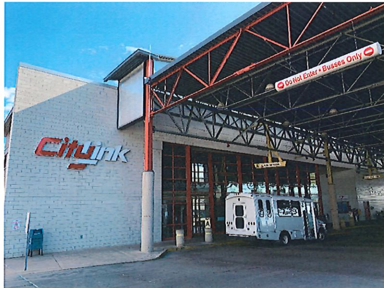
Transit Center – Passenger Transfer
