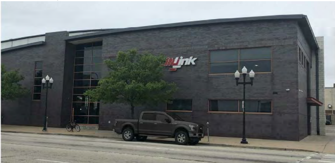
Transit Center – Passenger Transfer
