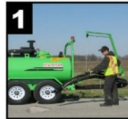
1 Clean area with on-board airstream.
