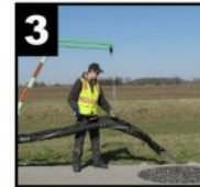
3 Apply aggregate/emulsion mixture - you're done!
