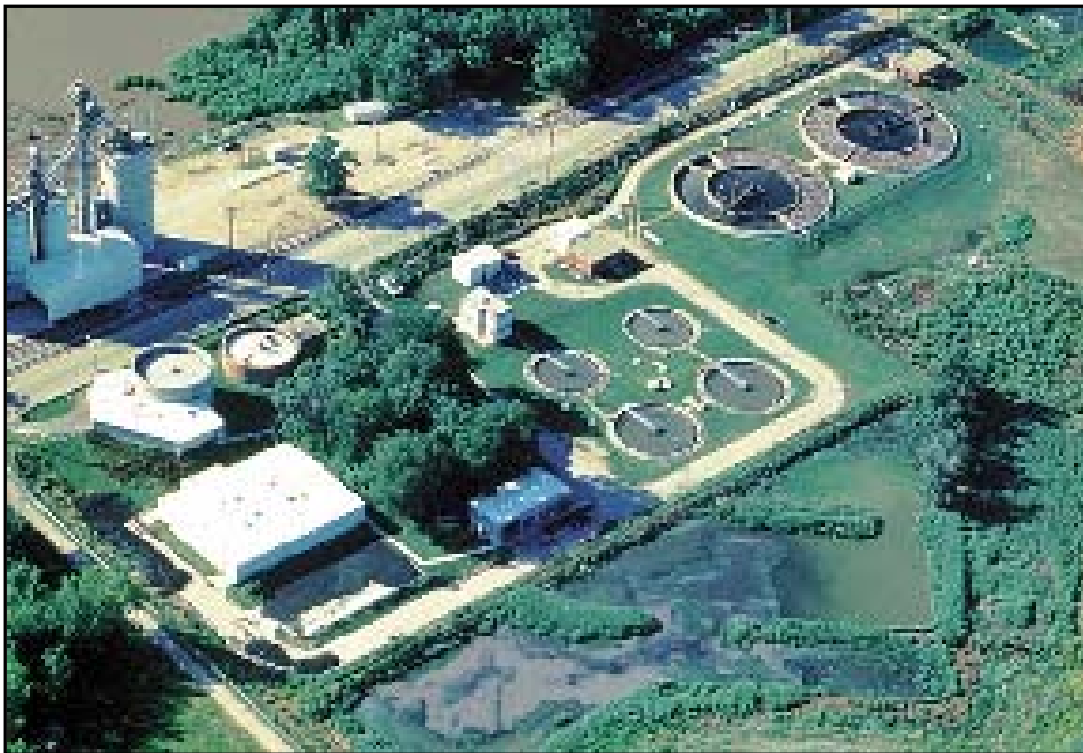
Pekin Wastewater Treatment Facility
