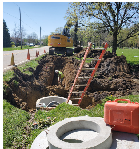
Metamora Storm Sewer Improvements
