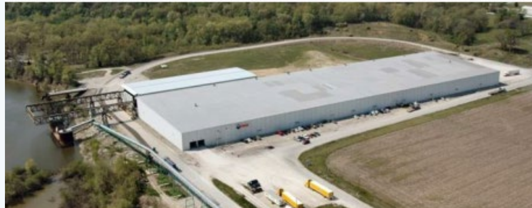
Example of Barge-Served Steel Plant at Kaskaskia
