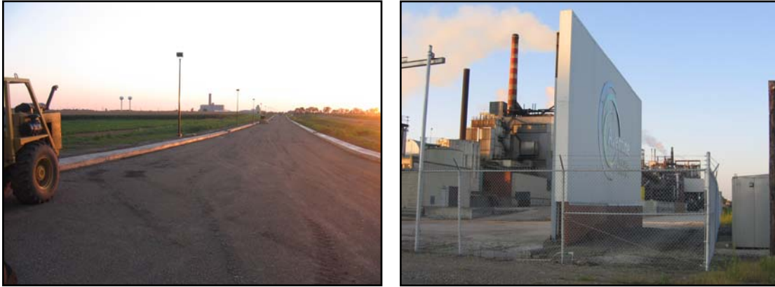
Figure 2. Additional infrastructure construction, such as the Hannah Drive extension pictured at left, will be required to facilitate new development in the South Industrial Area, and reinvestment in existing industrial operations (including the plants west of 2 nd Street, pictured at right), is needed to ensure the Area's continued economic viability.
