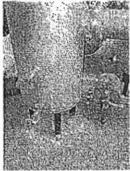
233 6" Condensate Sediment Traps w/ Sight glasses & Drip Traps
