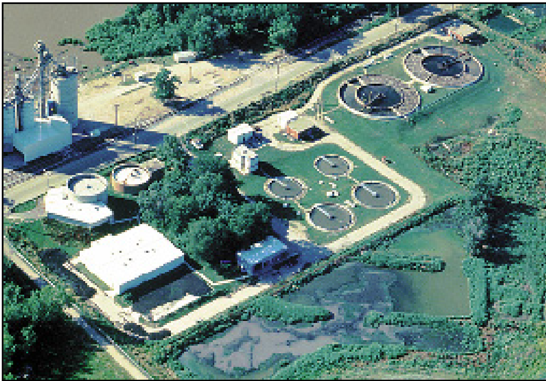
Pekin Wastewater Treatment Facility
