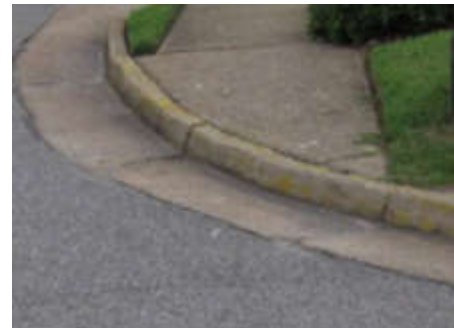
Sidewalk/Curb interface with missing ramp example. These locations were classified as a type of non-compliant curb ramp.
