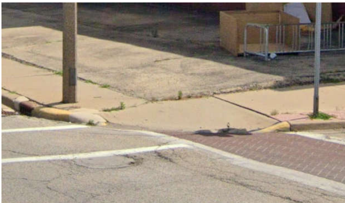
Curb Ramp example with adjacent painted cross walk. Also adjacent sidewalk obstruction.
