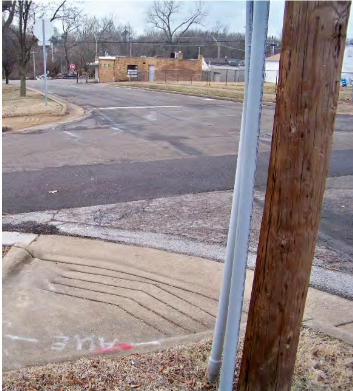
Existing Typical Ramp
