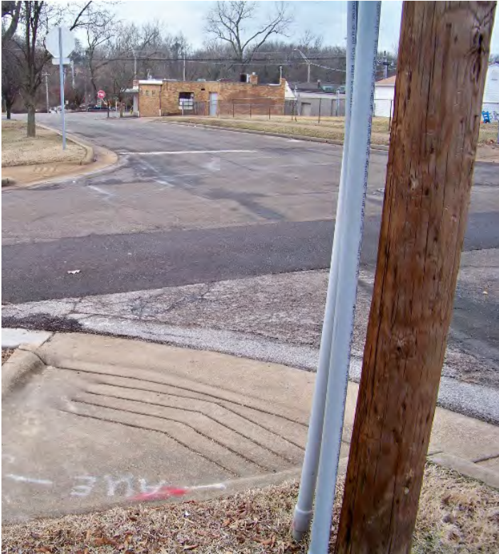
Existing Typical Ramp
