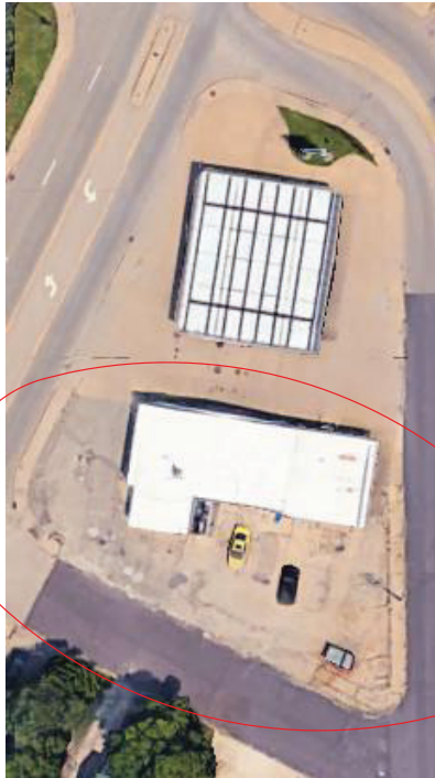
NEW ASPHALT BLACKTOP AT REAR AND SIDES OF BUILDING
