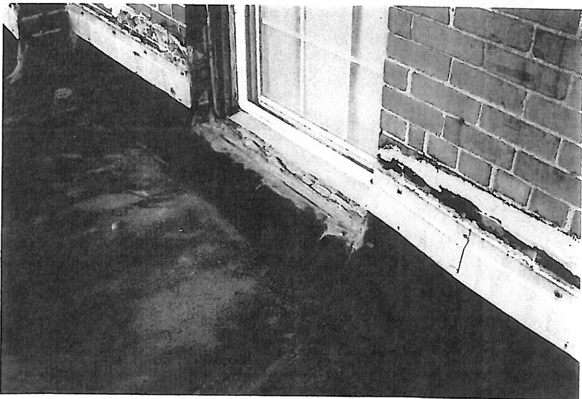
PHOTO NO. 18 - ROOF - WINDOW AT ADJACENT BUILDING
