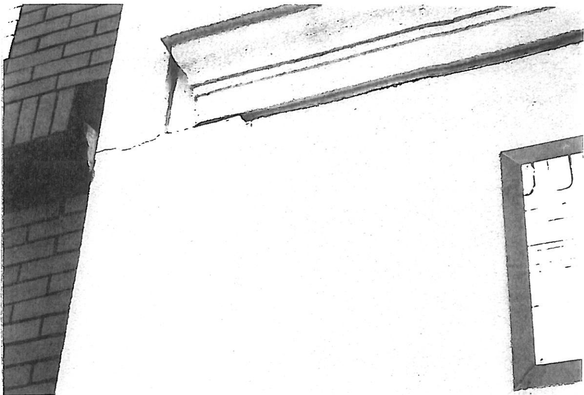
PHOTO NO. 2 - E.I.F.S. CRACKING AND DETERIORATED SEALANT JOINT
