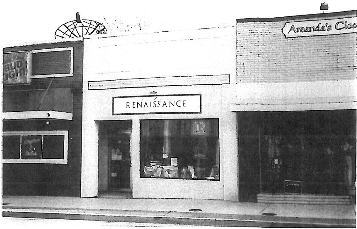
PHOTO NO. 1 - FRONT ( SOUTH) FACADE
