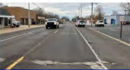
Typical roadway condition
