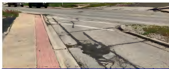
Typical sidewalk condition
