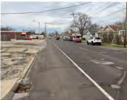
Example of filled curb face and inlet
