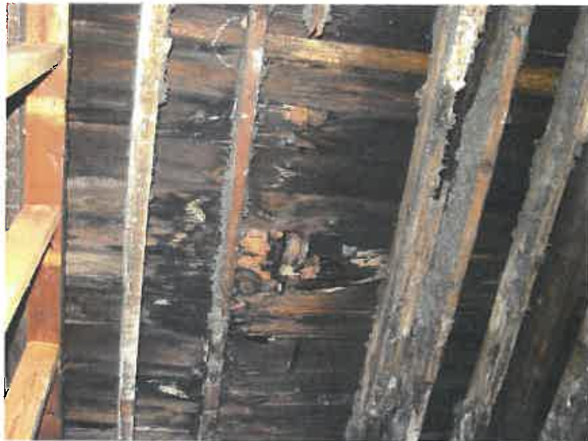
Image 11 (Roof Decking, Exposed Roof Membrane)
