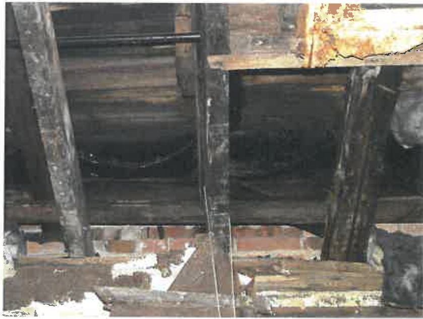
Image 10 (Roof Decking, Exposed Roof Membrane)
