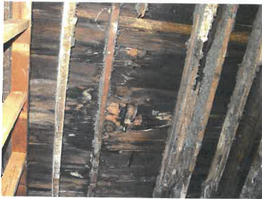
Image 11 (Roof Decking, Exposed Roof Membrane)
