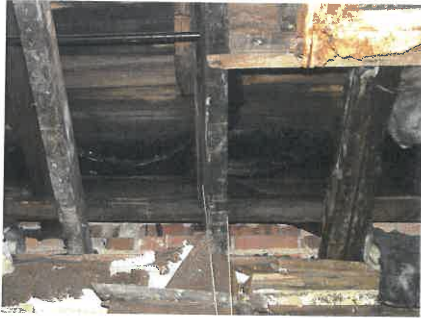
Image 10 (Roof Decking, Exposed Roof Membrane)
