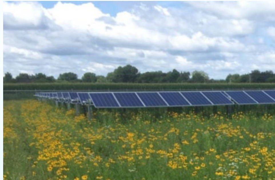
Example of single-axis tracker system in summer.
