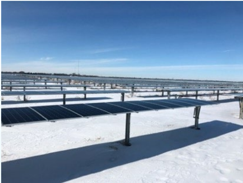
Single-axis tracker system in winter in Illinois.
