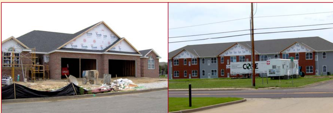
Duplex under construction on Remington Road; July 2007
