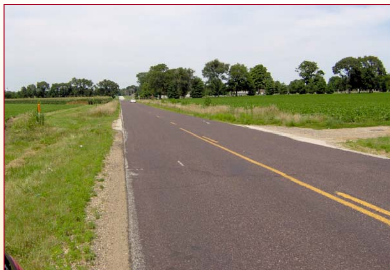
Typical topography. 5 th Street looking South
